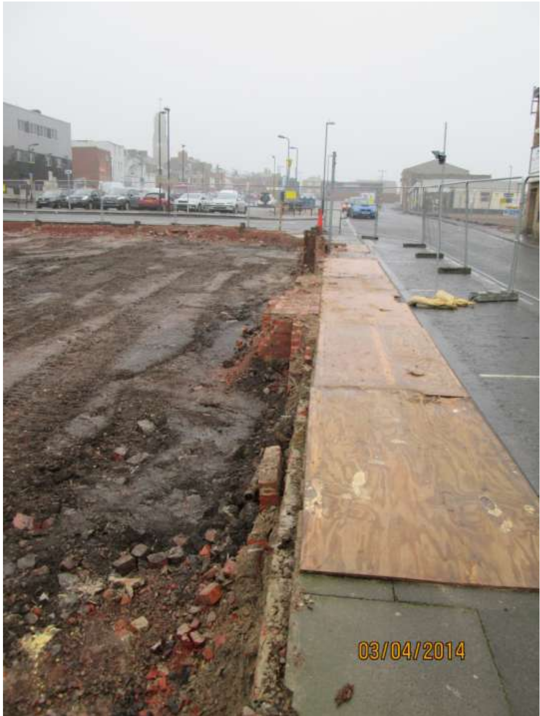
Foundations left in situ adjacent William St
