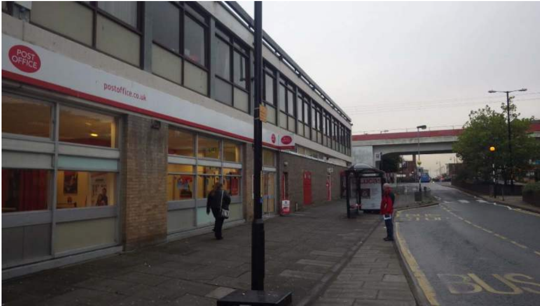
Photograph 1 Post Office Building. Facing West on Keppel Street.
