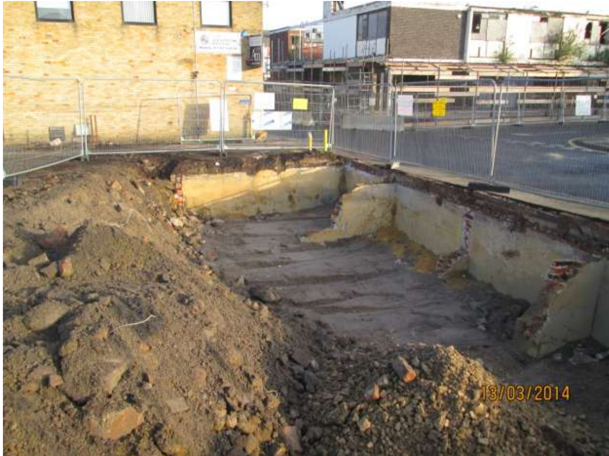
Foundations left in situ, adjacent William St
