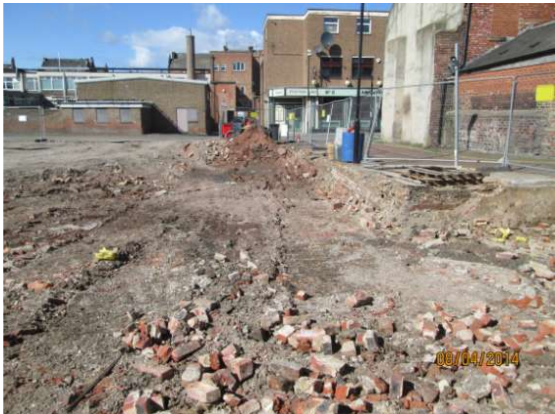
Foundations left in situ to Albermarle St and adjacent back lane
