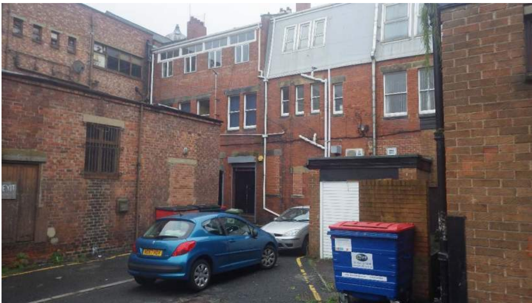
Photograph 2 Courtyard to rear of Keppel Street shops. Facing Northeast.
