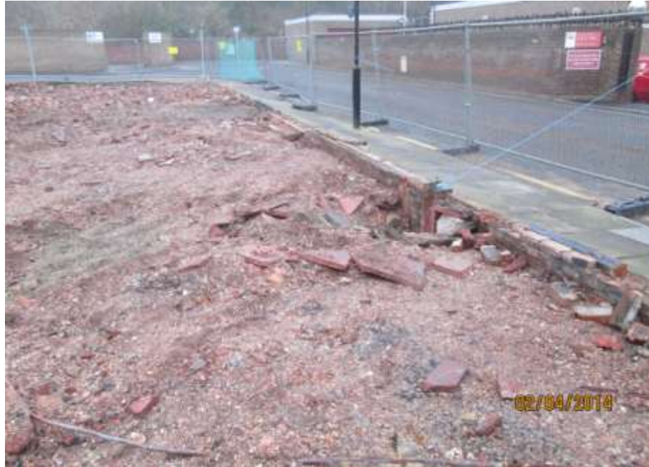
Foundations left in situ to Albermarle St and adjacent back lane
